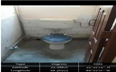
SINGLE TOILET BLOCK IN LADIES COMMON ROOM
