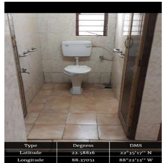
TOILET FOR PHYSICALLY HANDICAPPED
